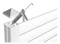
Close the top of the post with an end cap with screws or two-component epoxy glue.
