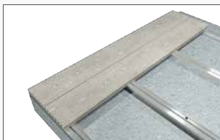
7) Installation of two slats
