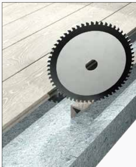
1) Cut all corner profile ends at 45 degrees
